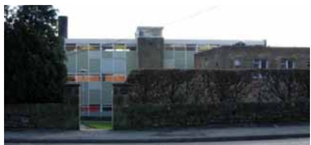
Below: mid twentieth century block on the Chatsworth Hall site
