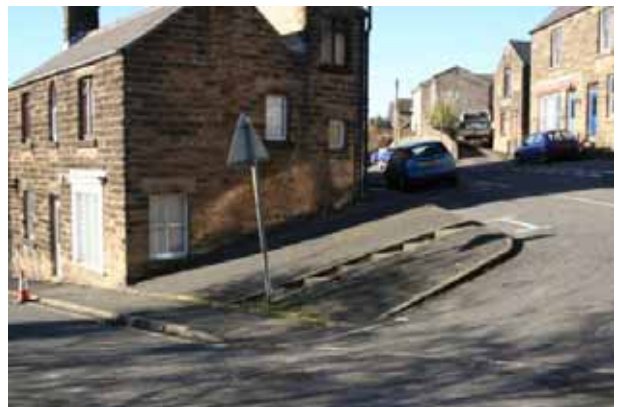
Corner of Jackson Road and Wellington Street
