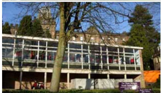
Above: two images of blocks obscuring the west wing of County Hall
