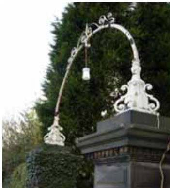
The arched wrought iron lantern holder at Chatsworth Hall (former hydro) adds great interest to the entrance. Features like this are worth keeping in good repair to avoid corrosion of the metal-work
