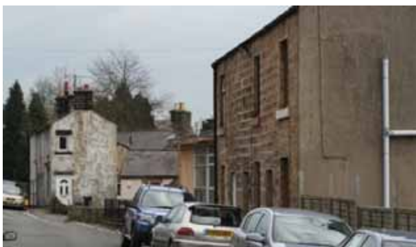
The neutral colour to render in the foreground is less visually obtrusive than the white render in the distance
