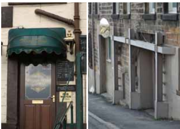
Above left: Features such as blinds, signs and light fittings, intended as ornamentation to facades, can become visual ‘clutter’ when used to excess.
